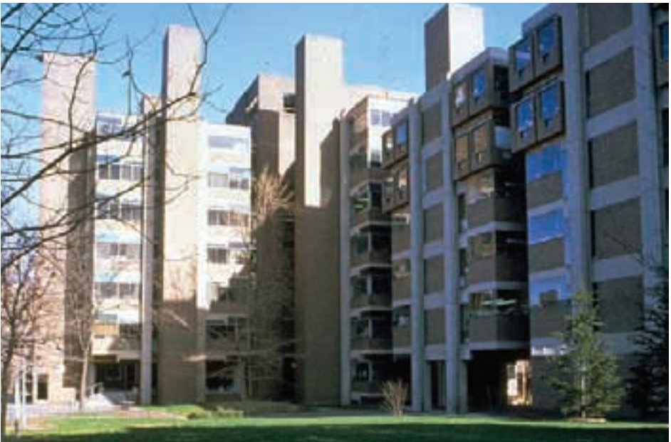
Figure 2: Richards Medical Research Building, University of Pennsylvania
