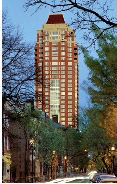
Figure 7: Symphony House, Philadelphia (Dranoff Properties, developer; BLT Architects).
