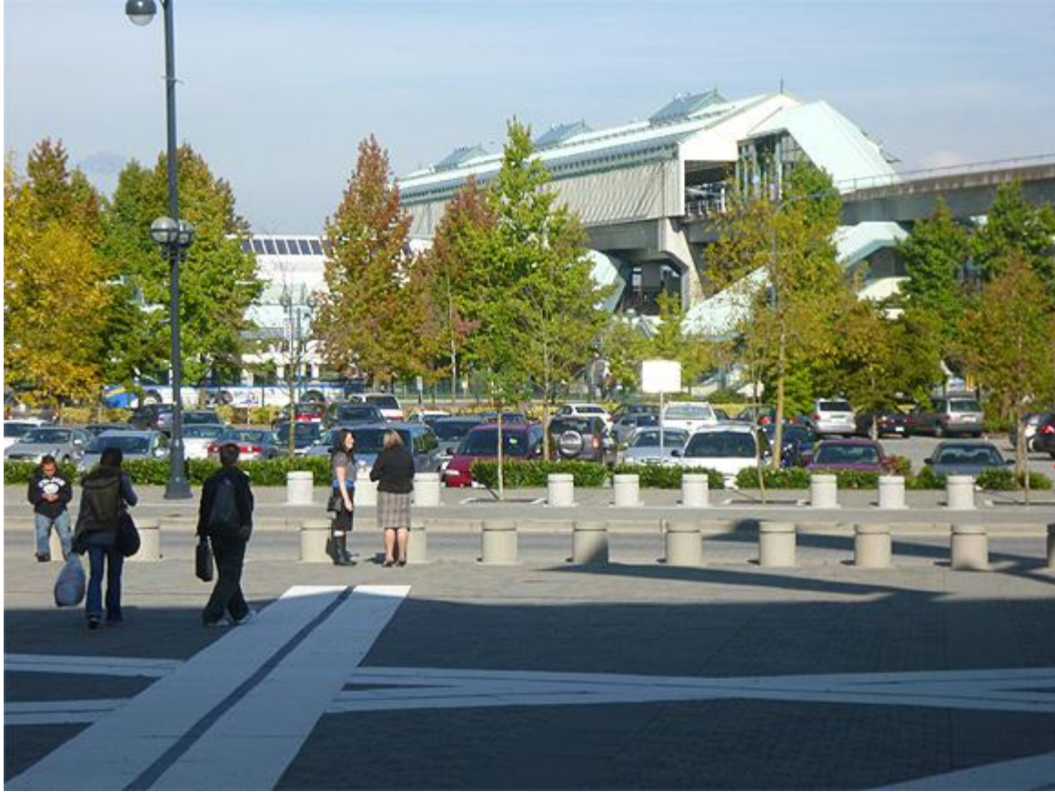
Figure 1: Skytrain station in Whalley.
